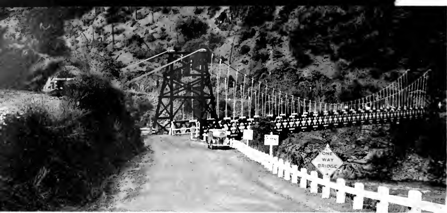
Feather River Bridge near Auburn built in 1929, a 322-foot suspension span with steel cables resting in saddles supported by timber A-frame towers which became unsafe due to dry rot and decay in towers
